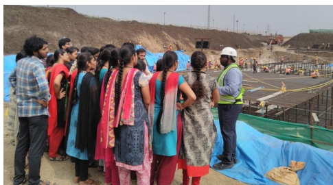
3/4 B.Tech students visited Amaravati High Court, Engineer Explaining about the foundation
