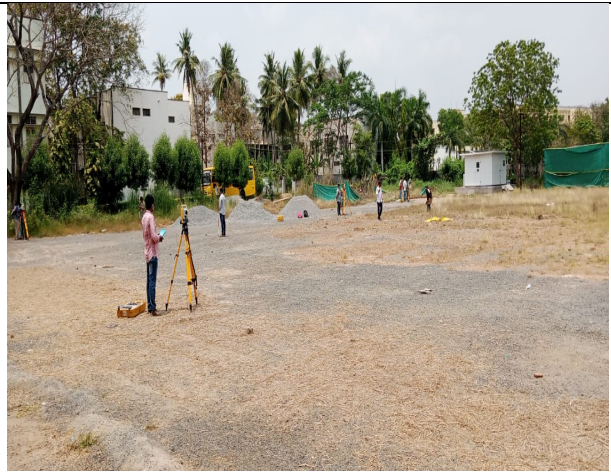
Survey Field Work
