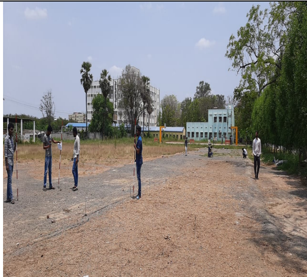
Survey Field Work
