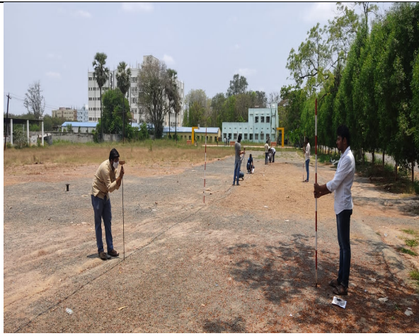
Survey Field Work
