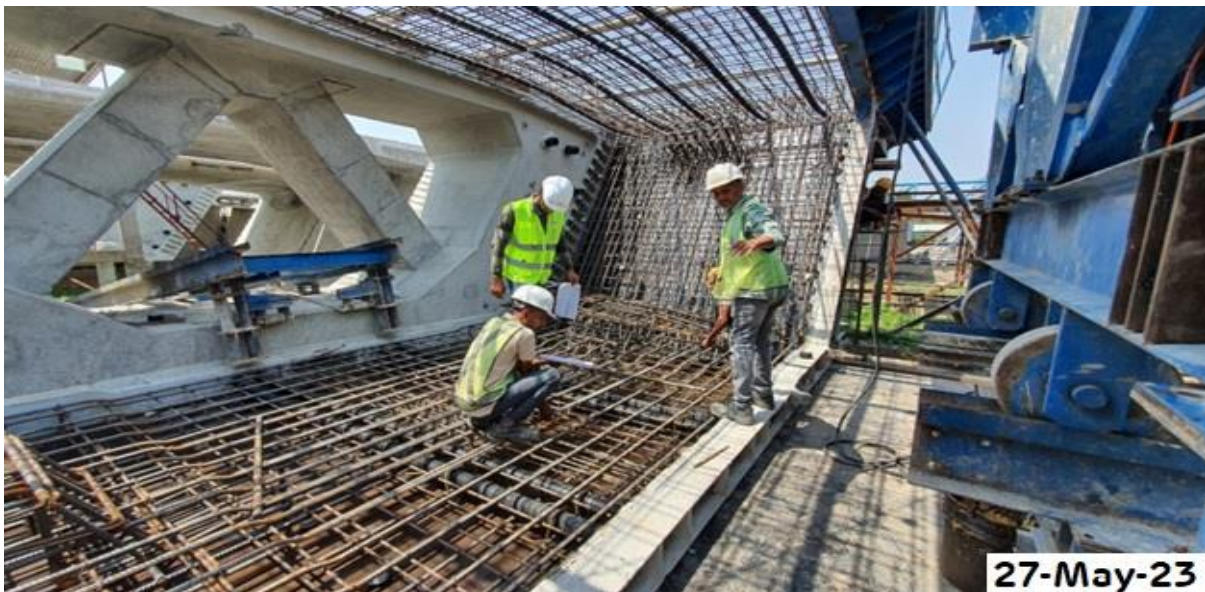
Fig.4. Arrangement of reinforcement for casting of box girder
