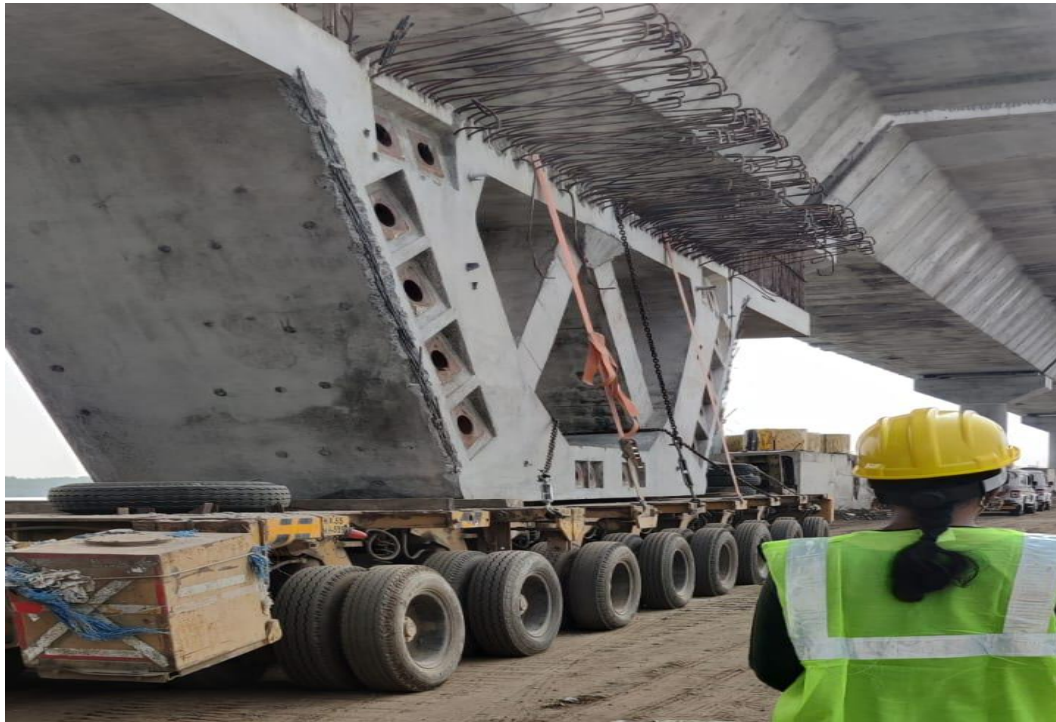
Fig.5. Shifting of girder from casting site to the location
