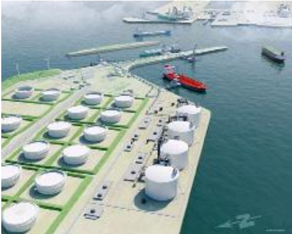
A large Liquefied Natural Gas (LNG) terminal.
